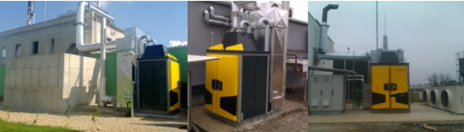
**ORC WB-I operates with flue gases within the range 350 - 520 °C. Thermal power at the input to the ORC WB-I is 450 - 900 kW while the electrical output power is 60 - 160 kW, depending on the input heat fed into the ORC system.**
